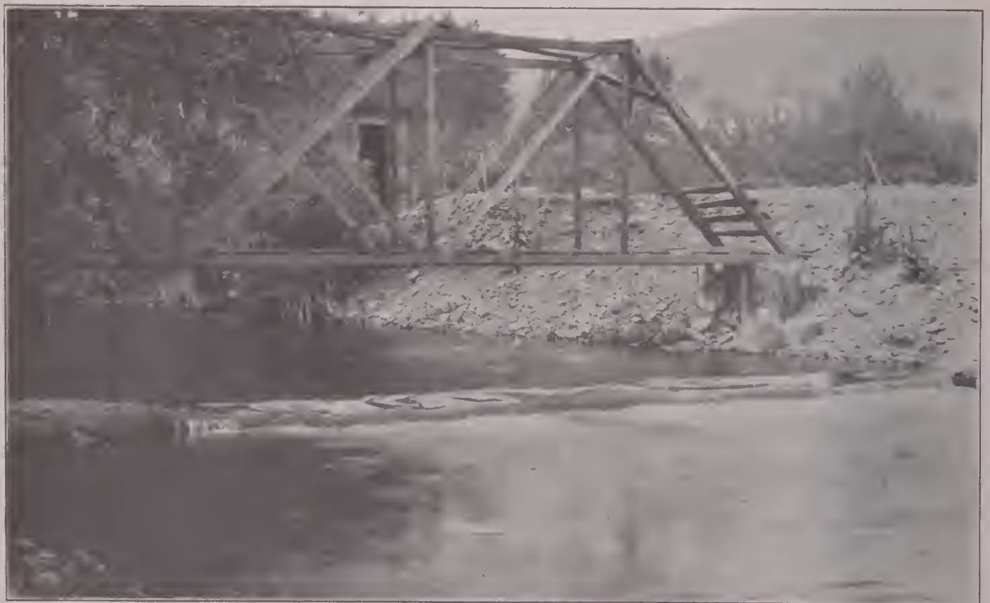
B. ARTIFICIAL CONCRETE CONTROL AND GAGING BRIDGE ON NORTH FORK OF AHTANUM CREEK NEAR TAMPICO.
